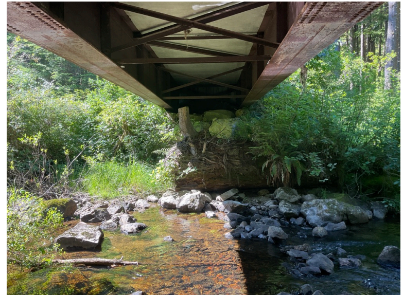
Left Bank Abutment when facing downstream
