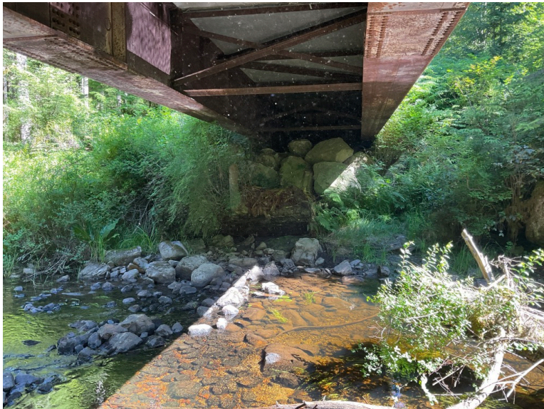
Right Bank Abutment when facing downstream
